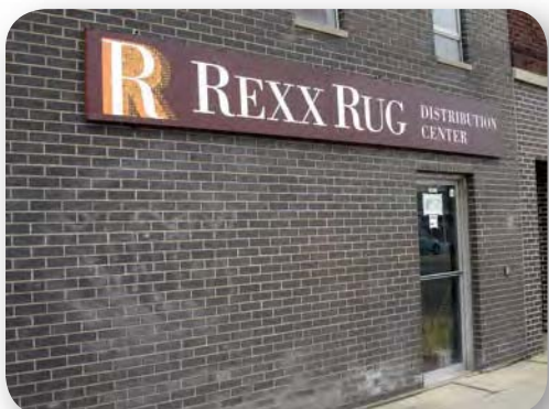
Aluminum panels mounted over entry door
